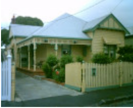
63 Clarence Street, Geelong West
