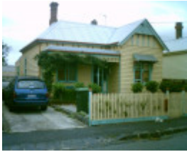
65 Clarence Street, Geelong West
