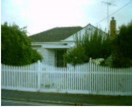
68 Clarence Street, Geelong West
