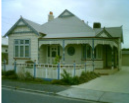
68a Clarence Street, Geelong West
