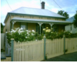
69 Clarence Street, Geelong West
