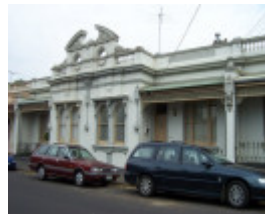
H01205 nathan s terrace 7 shield street flemington exterior2 feb2003
