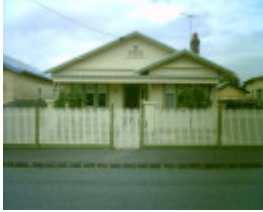
77 Clarence Street, Geelong West
