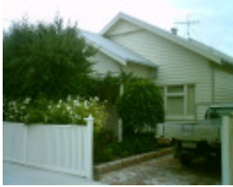
86 Clarence Street, Geelong West
