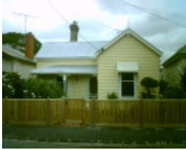
89 Clarence Street, Geelong West
