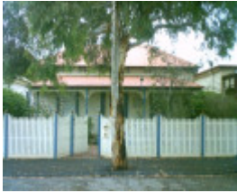
95 Clarence Street, Geelong West
