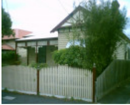
97 Clarence Street, Geelong West
