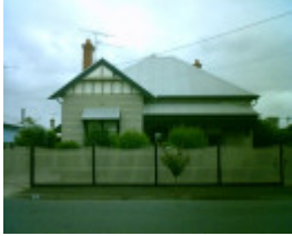
98 Clarence Street, Geelong West
