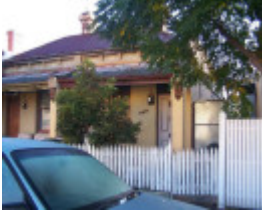
RICHMOND SOMERSET STREET 103.jpg
