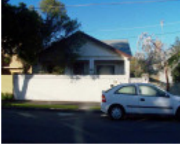
RICHMOND SOMERSET STREET 112.jpg
