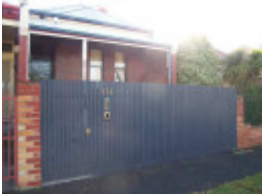
RICHMOND SOMERSET STREET 113.jpg
