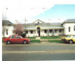
Alexandra court house
