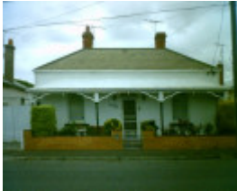
109 Clarence Street, Geelong West
