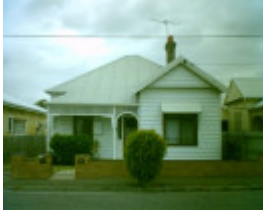
113 Clarence Street, Geelong West
