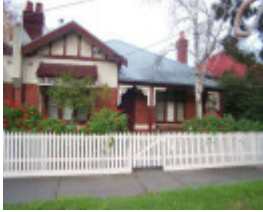
RICHMOND SOMERSET STREET 158.jpg
