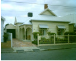
115 Clarence Street, Geelong West
