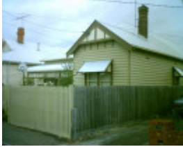
117 Clarence Street, Geelong West
