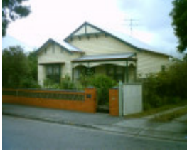
118 Clarence Street, Geelong West
