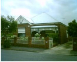
120 Clarence Street, Geelong West
