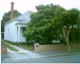
123 Clarence Street, Geelong West
