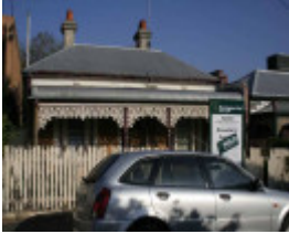
RICHMOND LESNEY STREET 14.jpg
