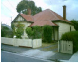
124 Clarence Street, Geelong West
