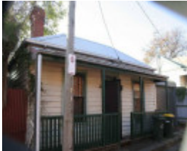
RICHMOND SHAMROCK STREET 9.jpg
