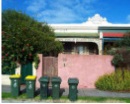
RICHMOND BAKER STREET 60.jpg
