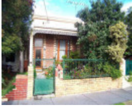
RICHMOND BAKER STREET 64.jpg
