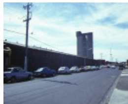
former melvilles grainstore colebrook street brunswick side elevation building 2
