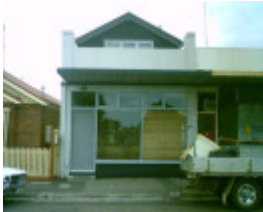
17a Elizabeth Street, Geelong West
