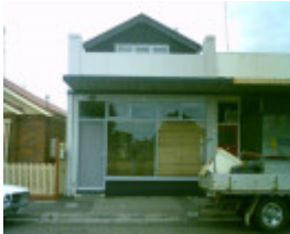
17a Elizabeth Street, Geelong West
