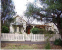
RICHMOND MURPHY STREET 14.jpg
