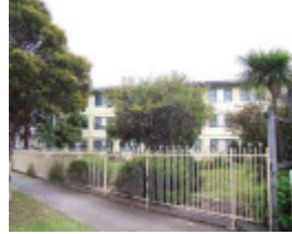
RICHMOND MURPHY STREET 17-21 Unit 15.jpg
