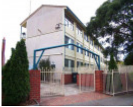
RICHMOND MURPHY STREET 17-21 Unit 1.jpg
