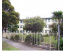
RICHMOND MURPHY STREET 17-21 Unit 15.jpg
