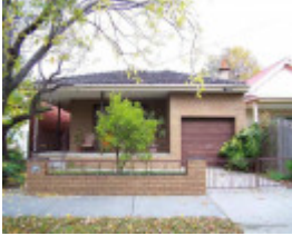
RICHMOND MURPHY STREET 26.jpg
