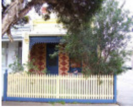
RICHMOND MURPHY STREET 27.jpg
