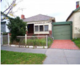
RICHMOND MURPHY STREET 32.jpg
