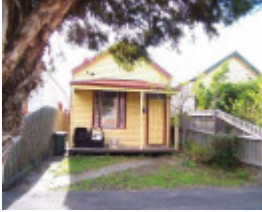
RICHMOND MURPHY STREET 33.jpg
