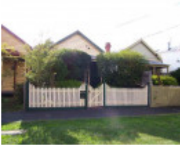
RICHMOND MURPHY STREET 35.jpg
