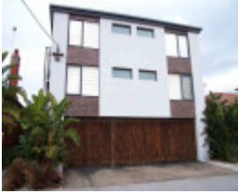
RICHMOND MURPHY STREET 42 Unit 1.jpg
