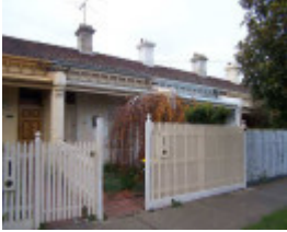
RICHMOND BURNLEY STREET 351.jpg
