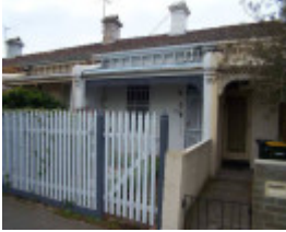
RICHMOND BURNLEY STREET 353.jpg
