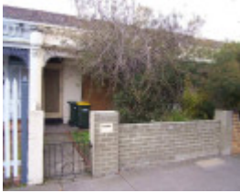
RICHMOND BURNLEY STREET 355.jpg
