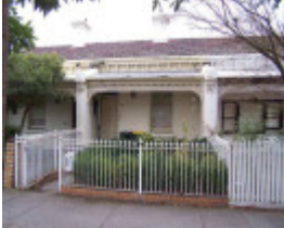
RICHMOND BURNLEY STREET 359.jpg
