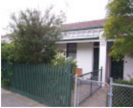
RICHMOND BURNLEY STREET 365.jpg
