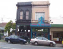
RICHMOND BURNLEY STREET 371.jpg
