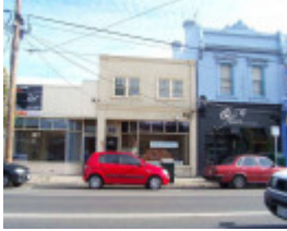
RICHMOND BURNLEY STREET 374.jpg
