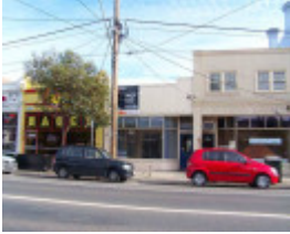
RICHMOND BURNLEY STREET 376.jpg
