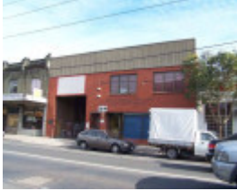
RICHMOND BURNLEY STREET 382-386.jpg
