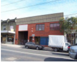
RICHMOND BURNLEY STREET 382-386.jpg
