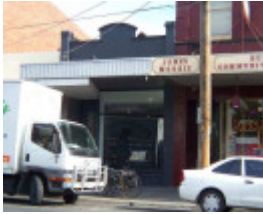
RICHMOND BURNLEY STREET 396.jpg
